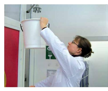
Labour-intensive water exchange at every terminal tapping point. A common, but ineffective and expensive solution to ensure proper operation in a building.
